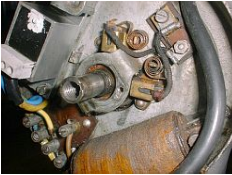
The PCB will be fitted by the help of a spacer.
